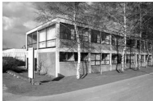
Herbert Hirche designed this Wilkhahn office building, built in 1960.
